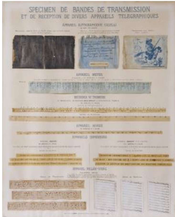
Fig. 9. Specimen of outputs of different telegraphs, with pantelegraph images at top, 1867. © Musée des arts et métiers-CNAM, Paris/Pascal Faligot
